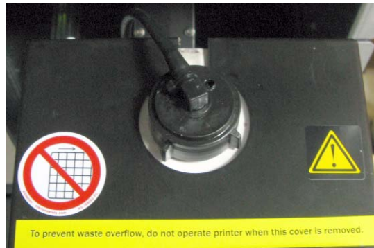
Figure 6-111: Fireproof cover installed over the waste container
